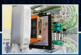
The MCC uses cutting-edge I/O-Link components to transmit crucial information, for example about availability and reasons for failure, or current feed forces.
